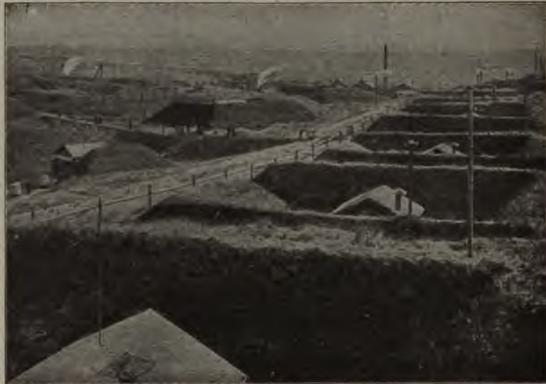
FACTORY FOR HIGH EXPLOSIVES, SHOWING EARTHEN WALLS, TO PROTECT AGAINST DISASTERS.
